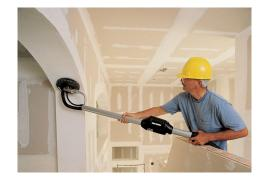
The Hook and Loop system for attaching abrasive paper to the foam backing is preferred by many. It is faster to change discs and it is more economical than the adhesive method. It also provides maximum adherence and a smooth, level sanding surface.
